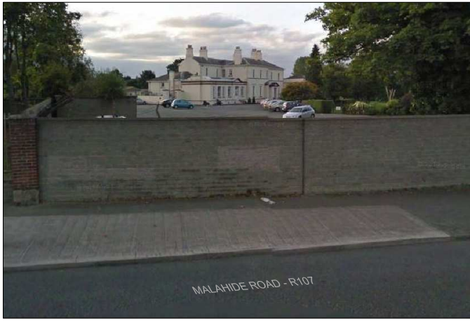
ESD VALVE 2 ENCLOSURE LOCATION EXISTING VIEW (NTS)
