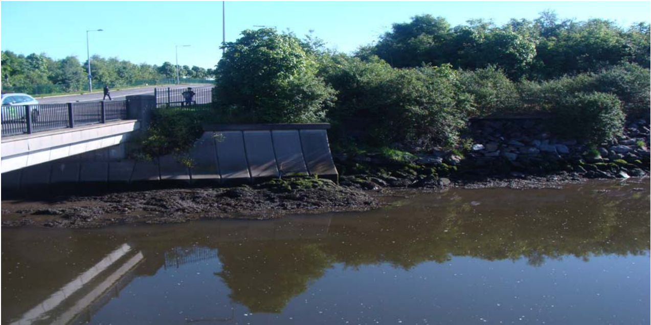
Figure 16.13: Tolka River in vicinity of crossing, looking north
