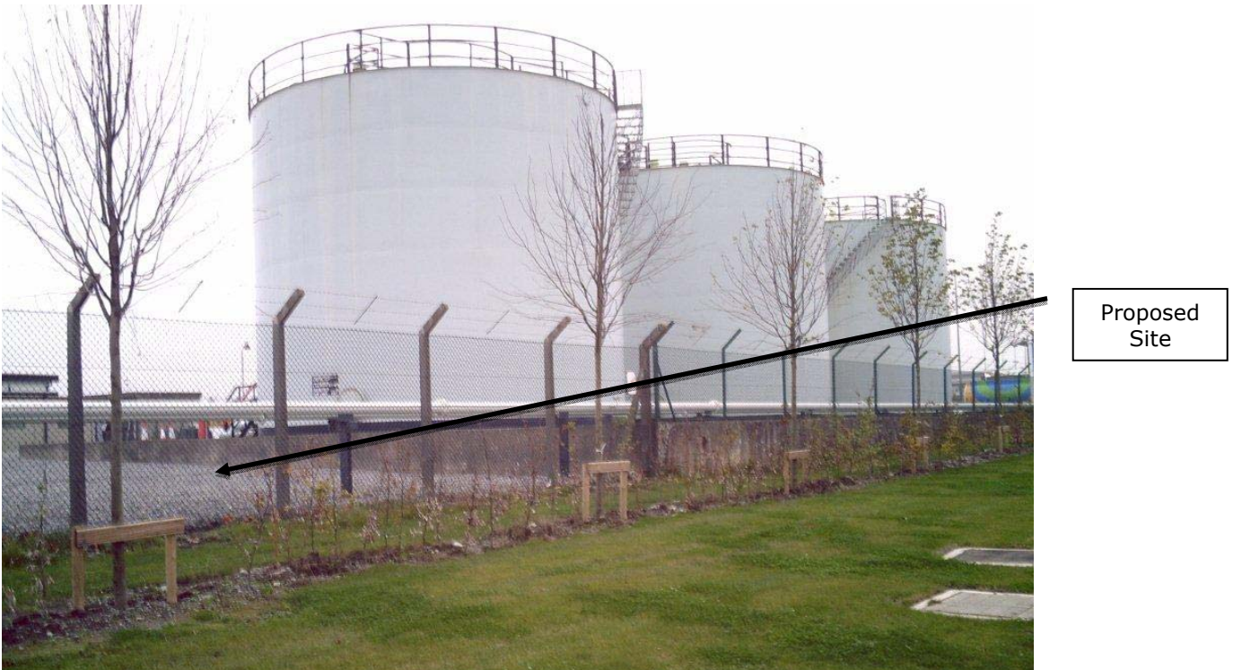
Figure 16.16: Reception Station at Dublin Airport
