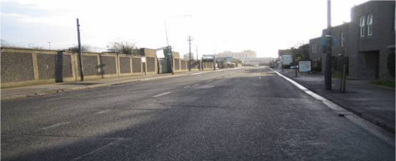
Figure 16.2: East Wall Road Looking south east
