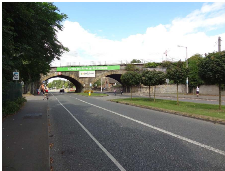
Figure 9.2: Clontarf Road Looking West (along westbound carriageway to rail bridge)
