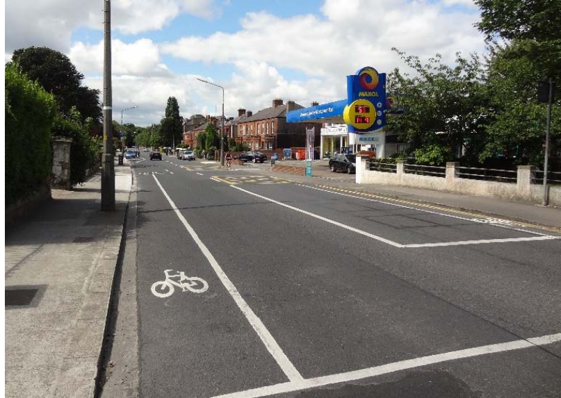
Figure 9.3: Howth Road Looking South (taken near Junction with Copeland Av)
